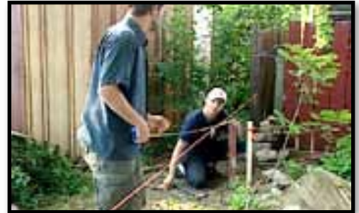
A. Laying out the fence line.
