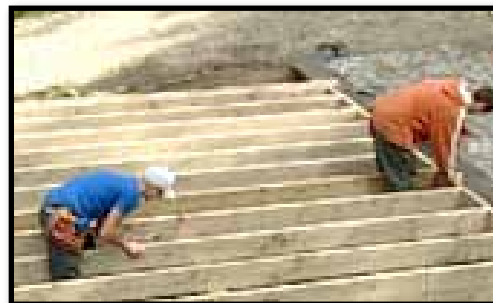
G. Setting the deck joists.
