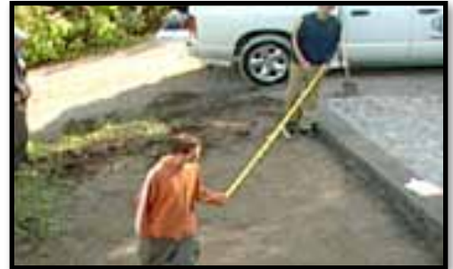
A. Laying out the deck plan.
