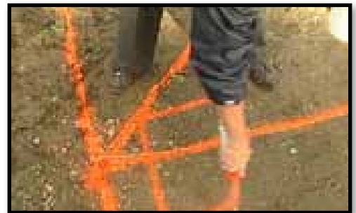
B. Using spray paint to outline the layout.
