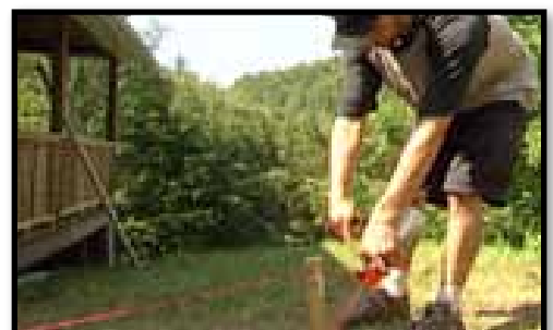
D. Using spray paint to mark the layout.
