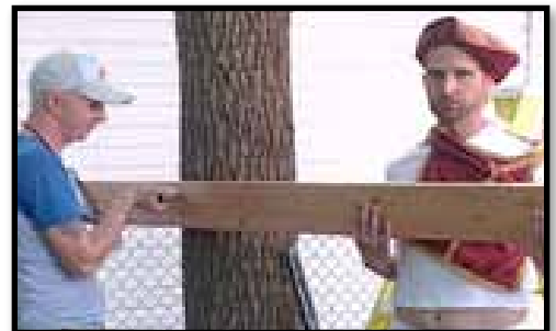
B. Bolting central support joists to tree.
