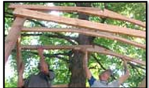
F. Installing rafters.
