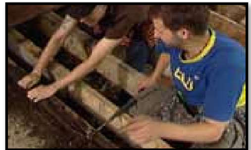
E. Replacing water damaged boards.
