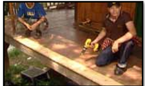
C. Replacing a porch board.
