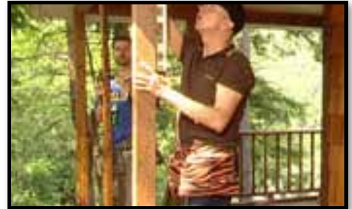
D. Replacing a support post.
