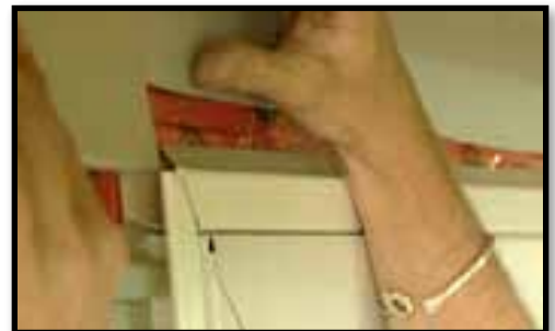
F. Siding over top of windows.
