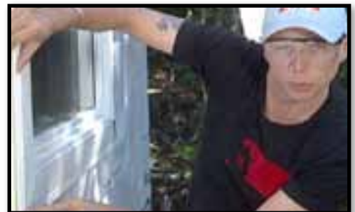
C. Installing J-channels.
