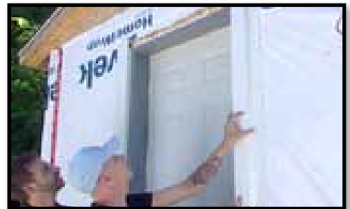
B. Installing flashing.
