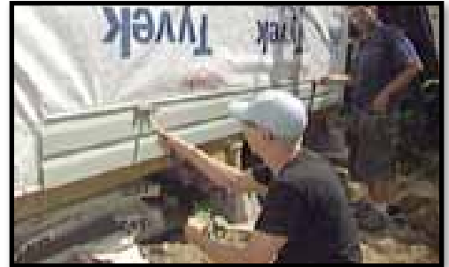
E. Installing the first full piece of siding.
