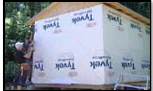
A. Putting up building paper.
