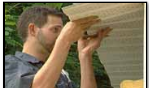
G. Installing soffit panels.
