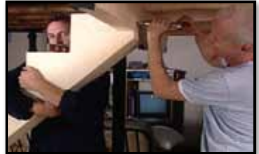
E. Attaching the stringer.
