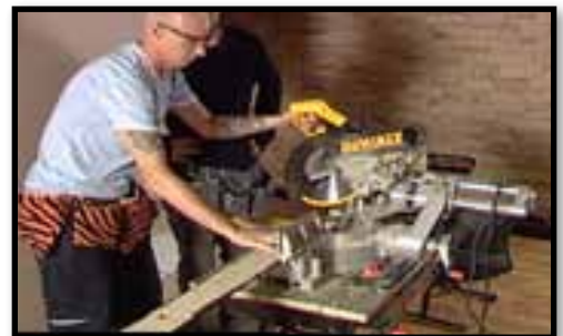
C. Installing decorative moulding.
