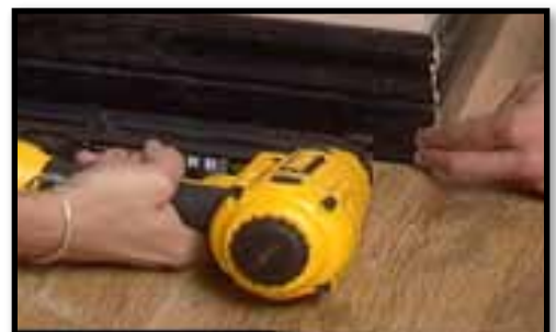
D. Installing baseboards.
