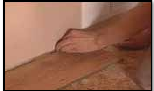
A. Spacers to create expansion gap.
