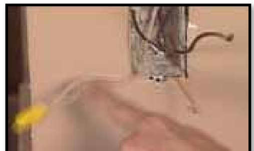
D. The white (neutral) wires are connected.
