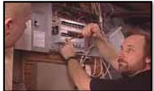
G. An electrician hooks up the breaker.
