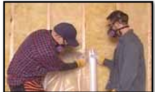
C. Installing a vapour barrier
