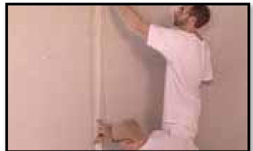
H. Put a layer of mud on the seems
