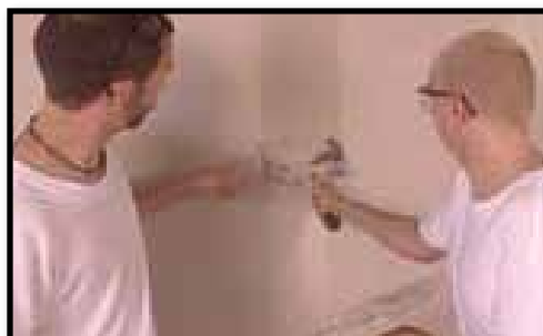
I. Apply drywall compound over the seams.
