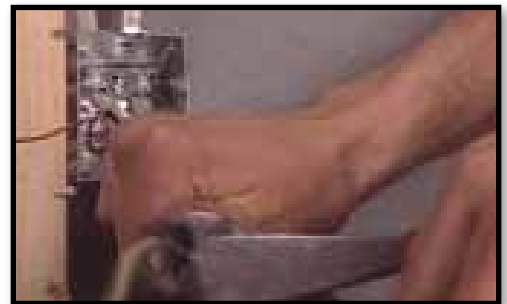
F. Strip the wire using a wire stripper.
