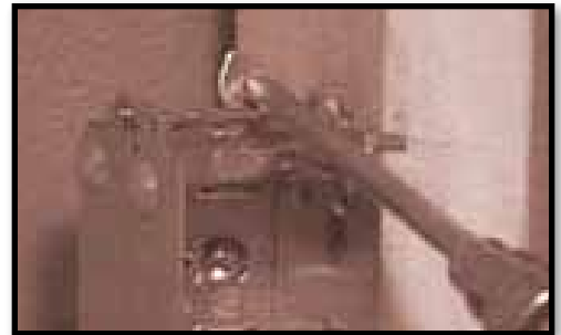
E. Knockout and feed the cable through.
