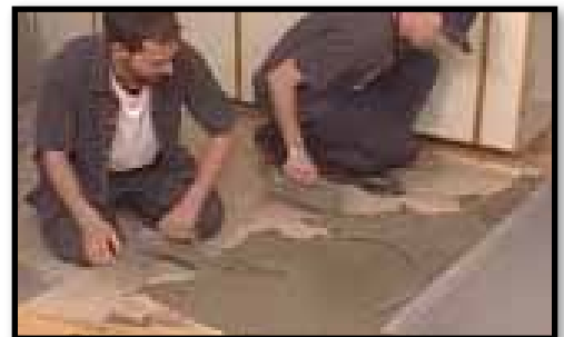
C. Applying extra thin mortar.
