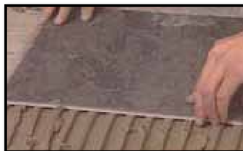
H. Gently twist the tile into place.
