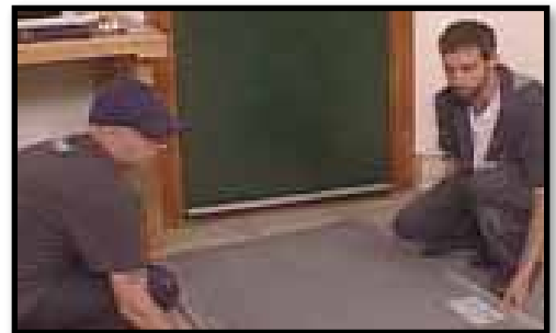
B. Layer of cement board.
