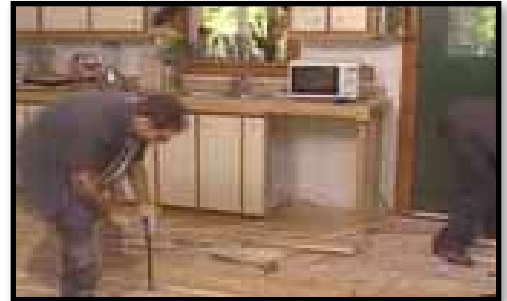
A. Removing the existing flooring.
