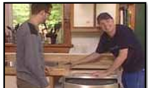
C. Measure the size of the dishwasher.
