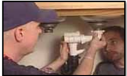
E. Inserting dishwasher and sink drain
