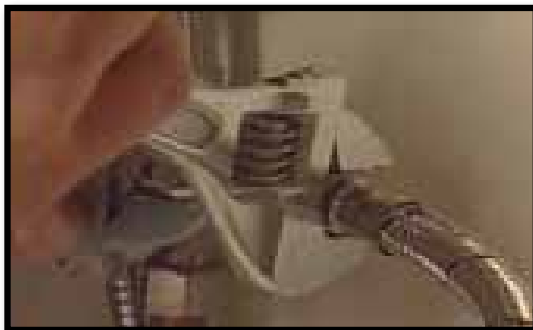
F. Hotwater feed off the t-junction
