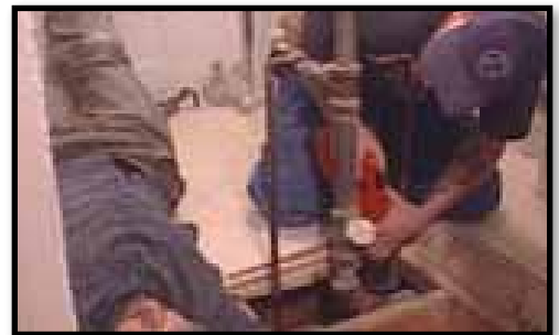
B. Removing old pipes w/ reciprocating saw.
