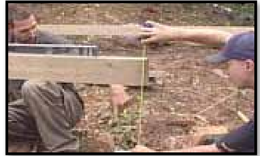
A. Levelling the Foundation.
