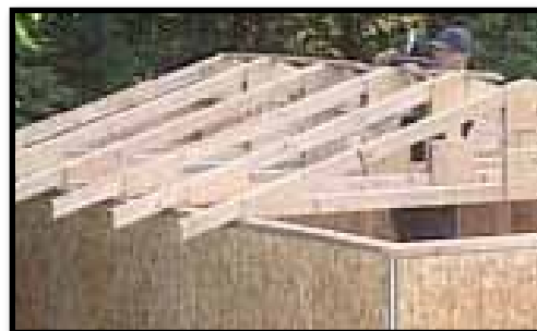
F. Installing the roof trusses.
