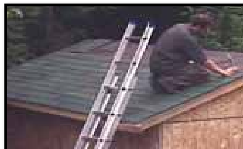
H. Installing the roof shingles.
