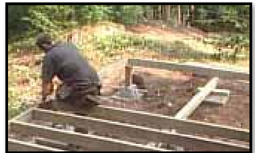
B. Building the Floor joists.
