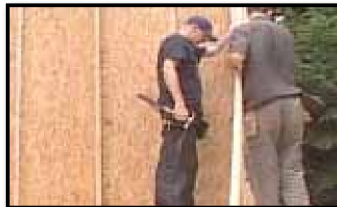
E. Bracing a wall.
